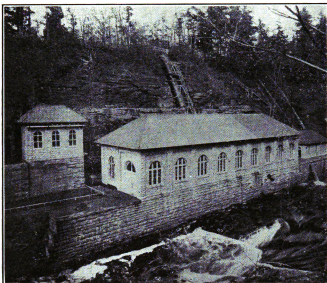
FIG. 93.—Trenton Falls Power House, Utica Gas & Electric Co.
